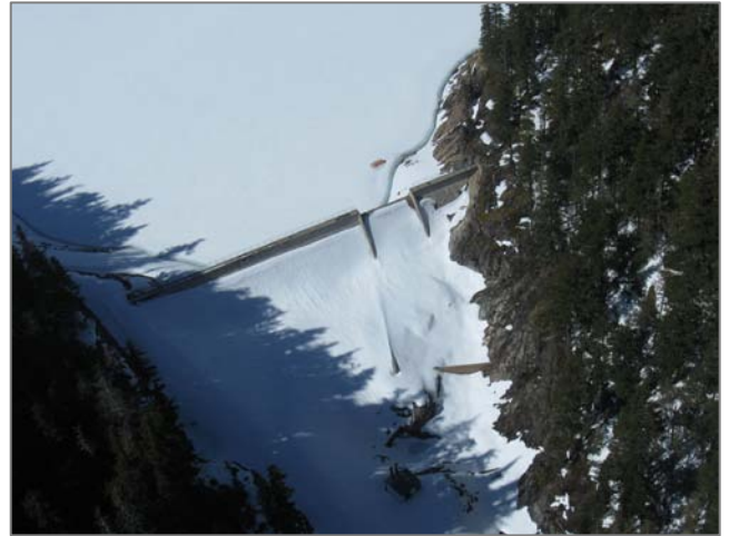
Arrowsmith Dam (April 2009)
