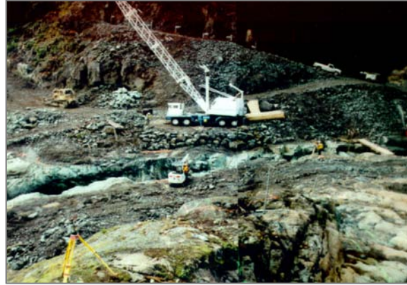
Arrowsmith Dam Construction 1998 - 1999
