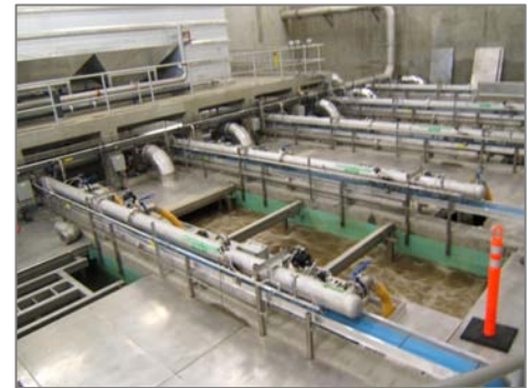
Water Treatment Facility – City of Kamloops
